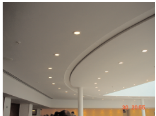
Coopers Smoke Curtain with curved 'all in one' ceiling interface
